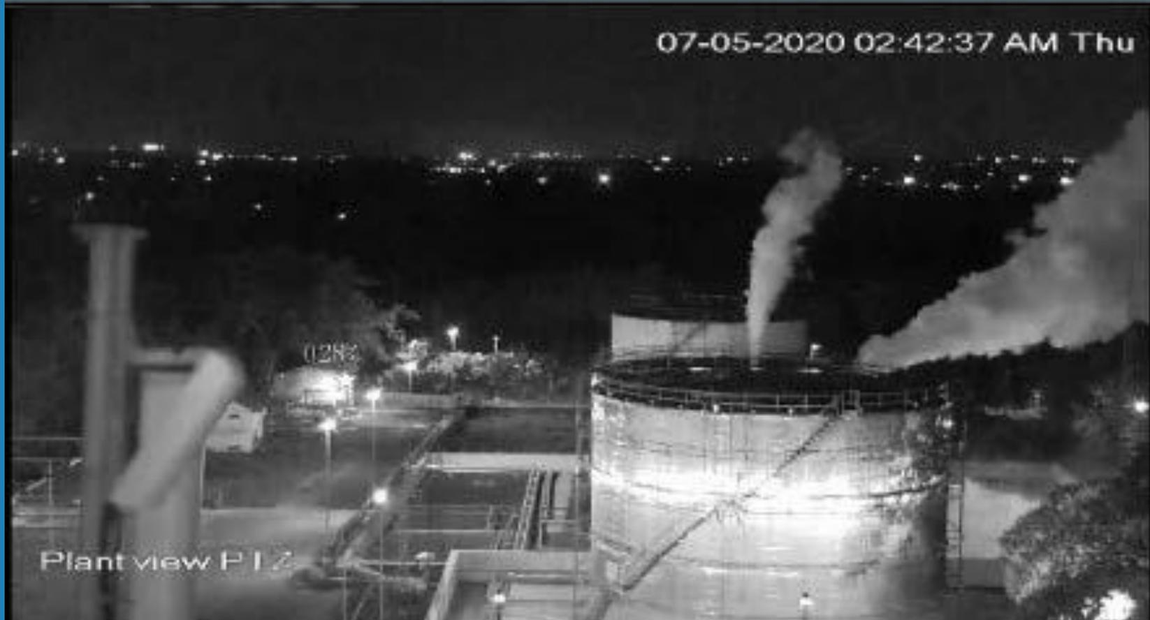
**Styrene Vapor Release from M6 Tank**
