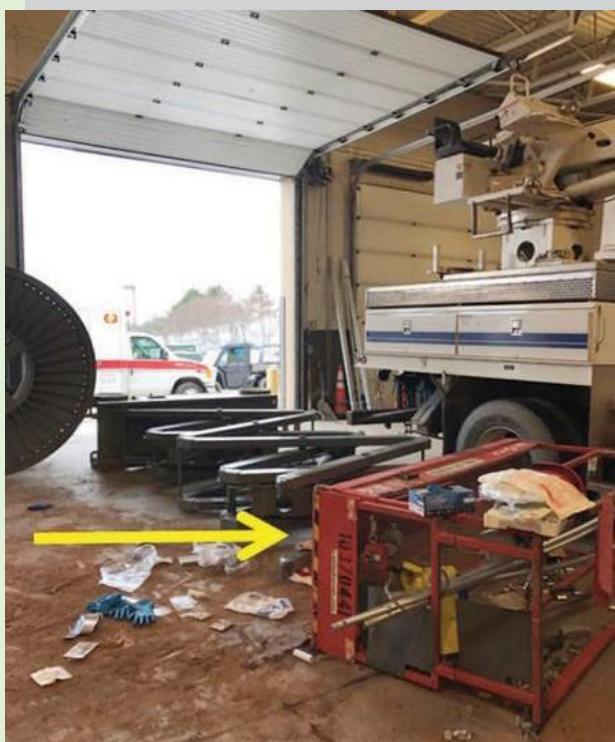
Photo 1: An electrician was working some 15 ft above the ground when an unknowing employee opened the garage door using a remote. As the door rose, it struck the lift and knocked it over.
