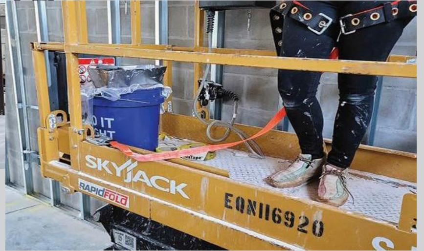
Photo 5 (below): The practice of requiring connection inside the scissor lift platform is controversial because it is not required by OSHA and because a worker who is tied off cannot escape if the lift tips over. Lift manufacturers warn that using the lanyard attachment anchorage as a fall arresting device could result in death or serious injury.
