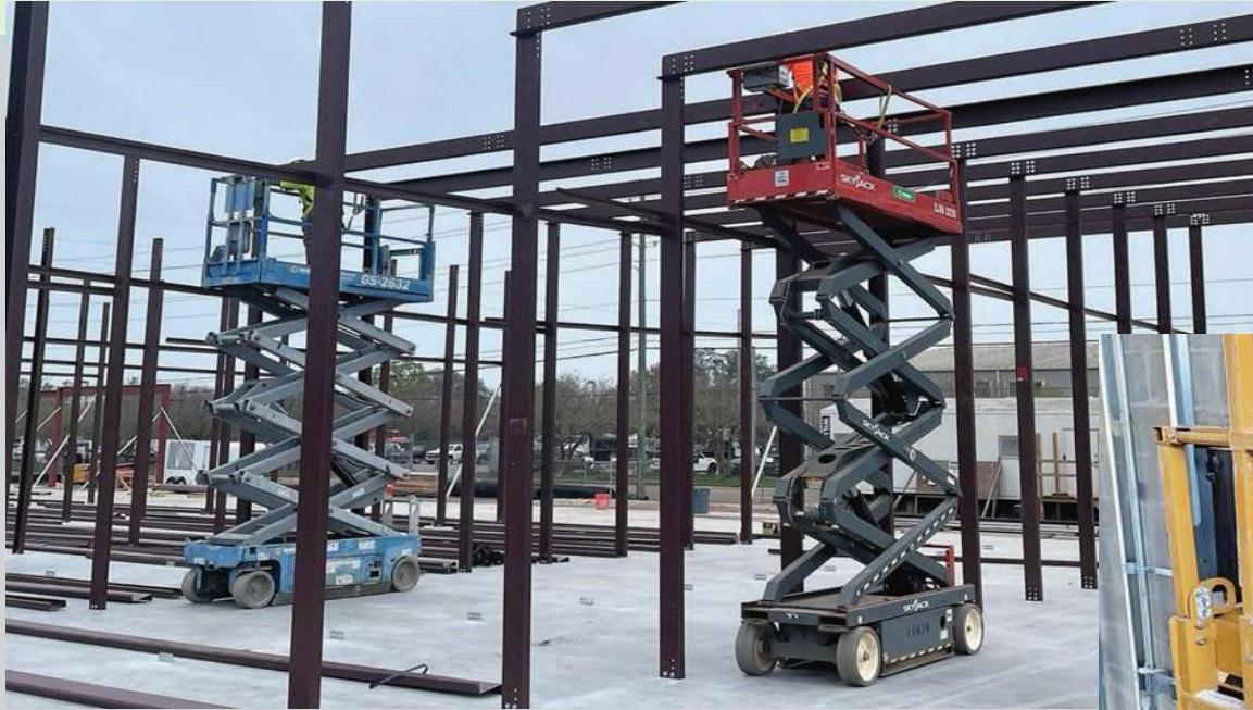
Photo 4 (above): Steel-erecting contractors using two parallel scissor lifts to place a beam across the handrails of both lifts—an extremely dangerous practice. Lift manufacturers specifically forbid the practice of using a scissor lift as a crane.
